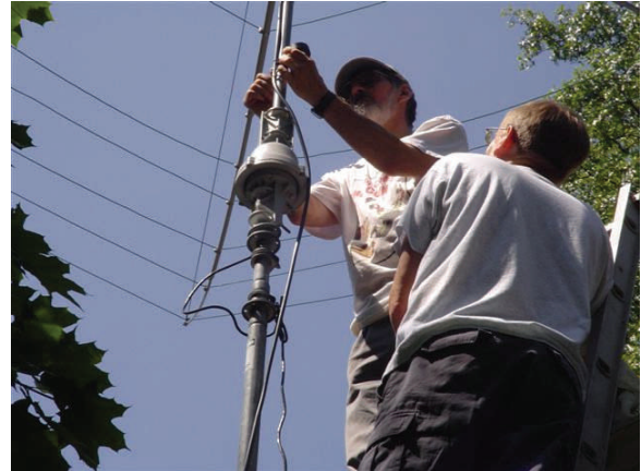
The intrepid roof crew
